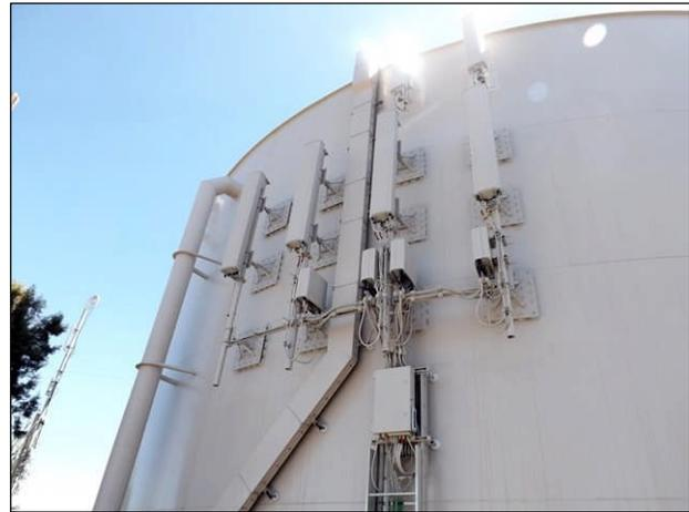
“Wind was the governing factor in this case,” said Al Di Donato, a structural engineer and owner of Di Donato Associates in San Diego, who recommended Magnemount. “Antennas are like sails in the wind. We have wind gusts here up to 80 miles per hour. They can shake the entire tank.” Taking that into consideration, Di Donato recommended the contractors install three magnetic plates for each antenna rather than the customary two plates.
